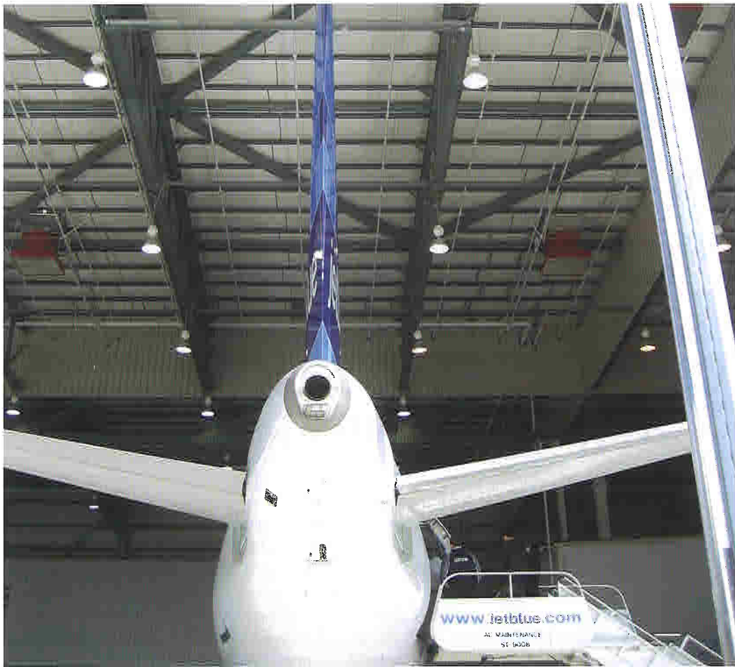
ALL The unique truss system allowed for maximum spans with a relatively shallow truss.
